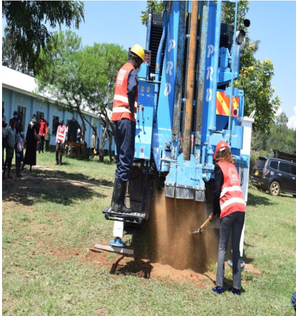
Plate 1: Borehole drilling
