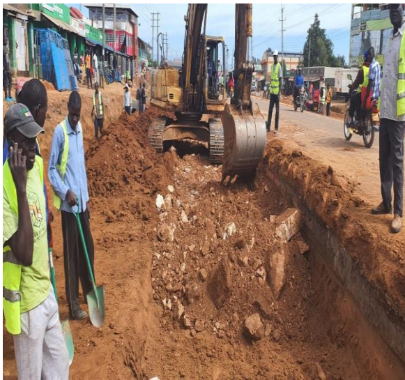
Plate 3: Upgrading of Musikoma- Kanduyi road- 6.5Kms
