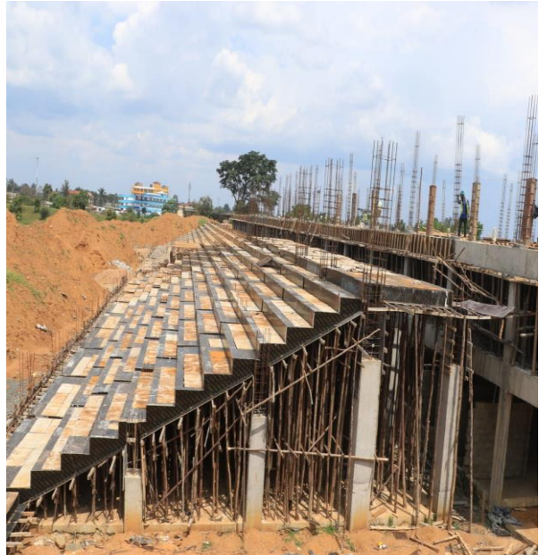
Plate 2: Modernization of Masinde Muliro stadium at Kanduyi
