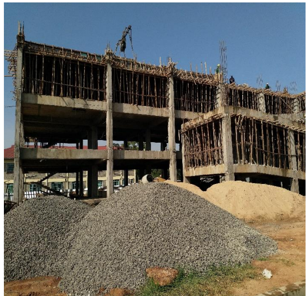
Plate 8: 300 bed capacity maternity under construction
