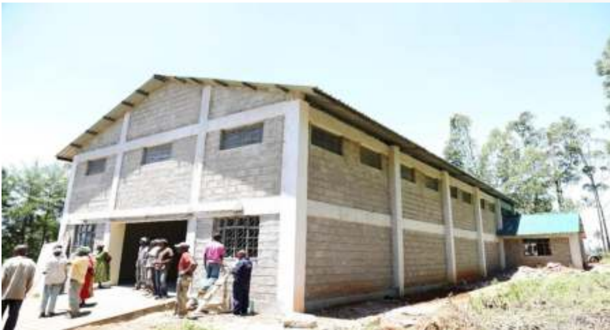
Figure 6: completed grain store in Kiminini
