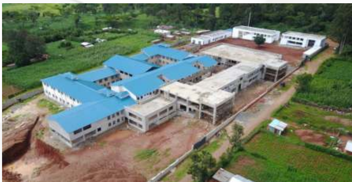
Figure 10: Trans Nzoia County Teaching and Referral Hospital at completion stages
