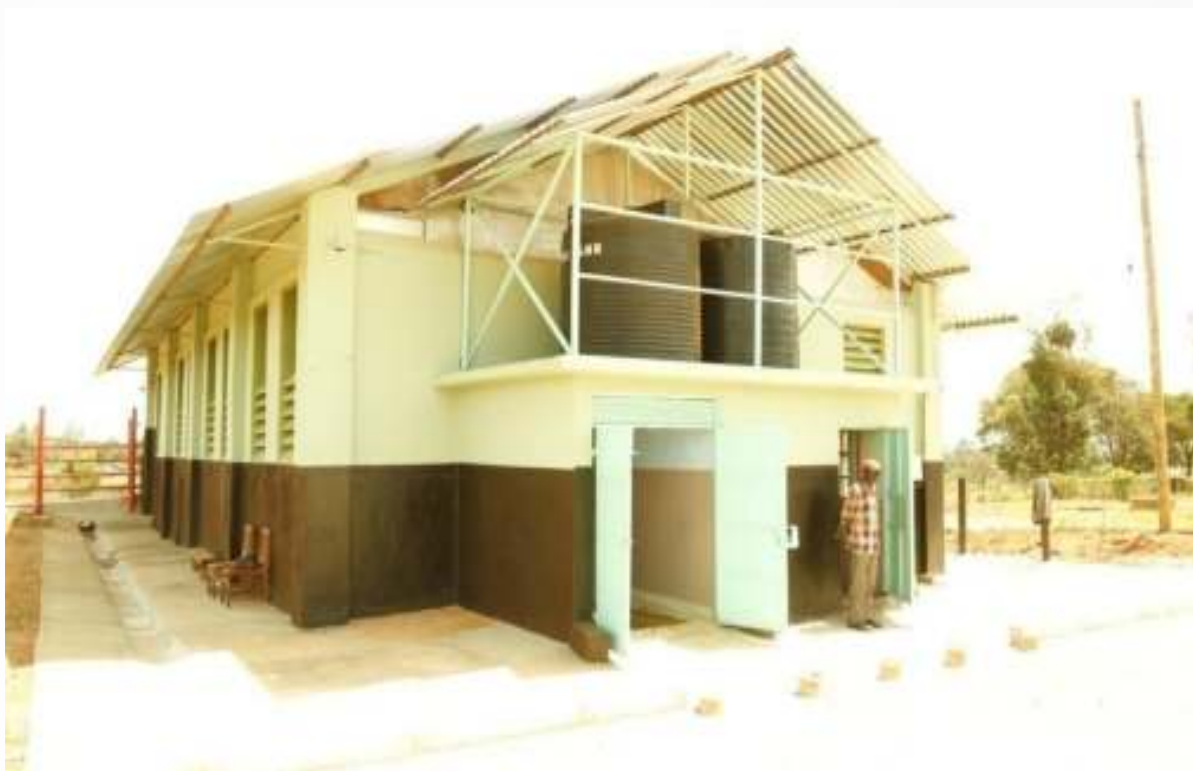
Figure 8: Renovated Machinjoni Slaughter House
