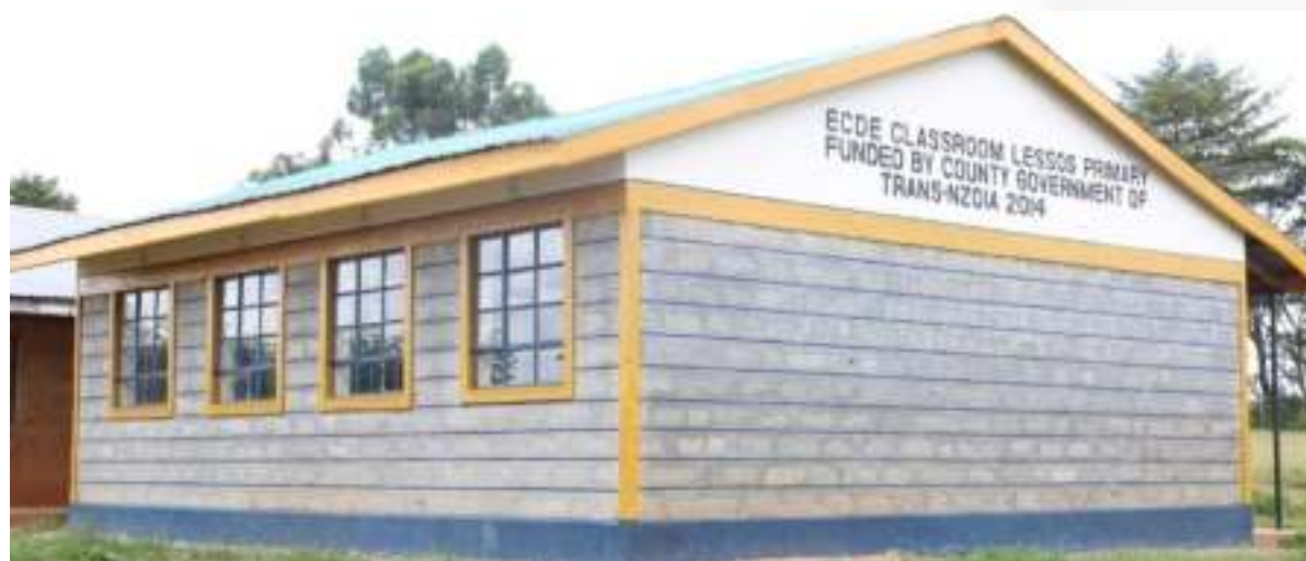
Figure 20: Completed ECDE classroom at Lessos Primary School
