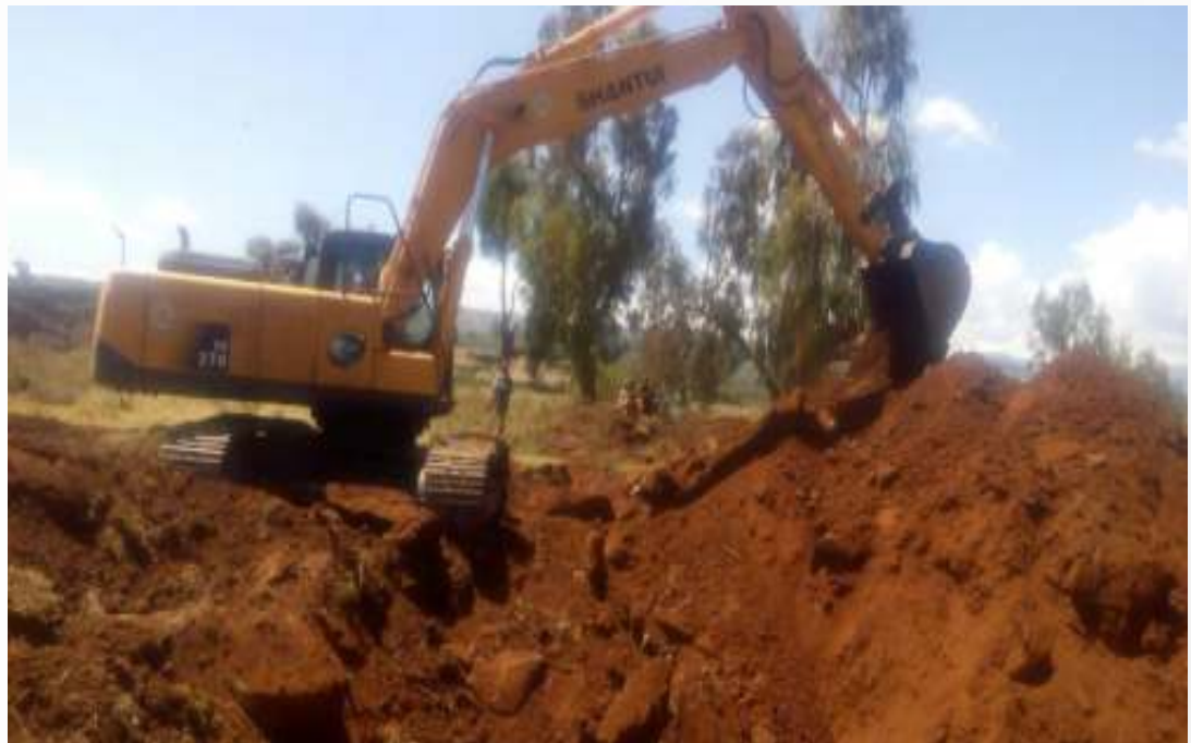
Figure 12: Excavation of murram at Chepchoina
