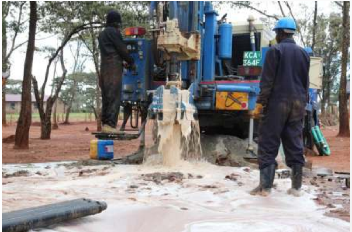
Figure 16: Water Drilling Rig at work
