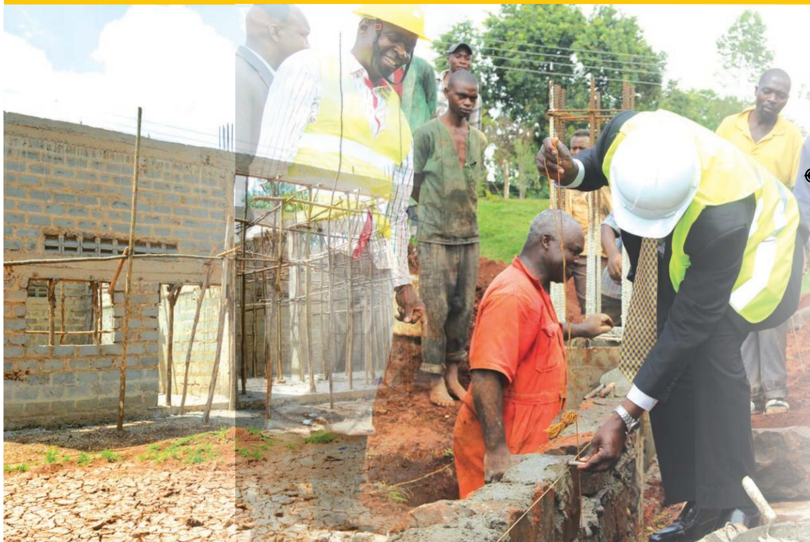
The Governor launching the Construction of Vihiga County Mechanical Unit
