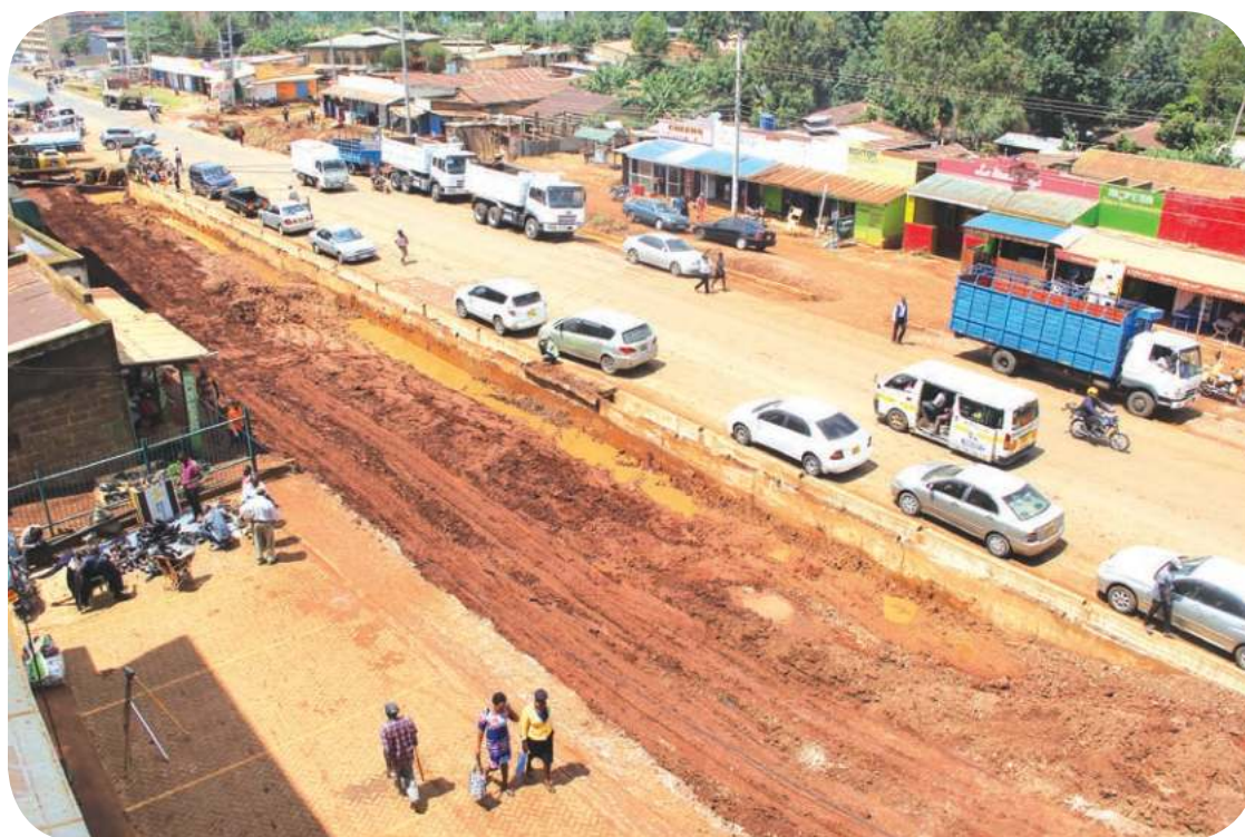
Mbale town urban facelift done by China Overseas Engineering Company (COVEC)
