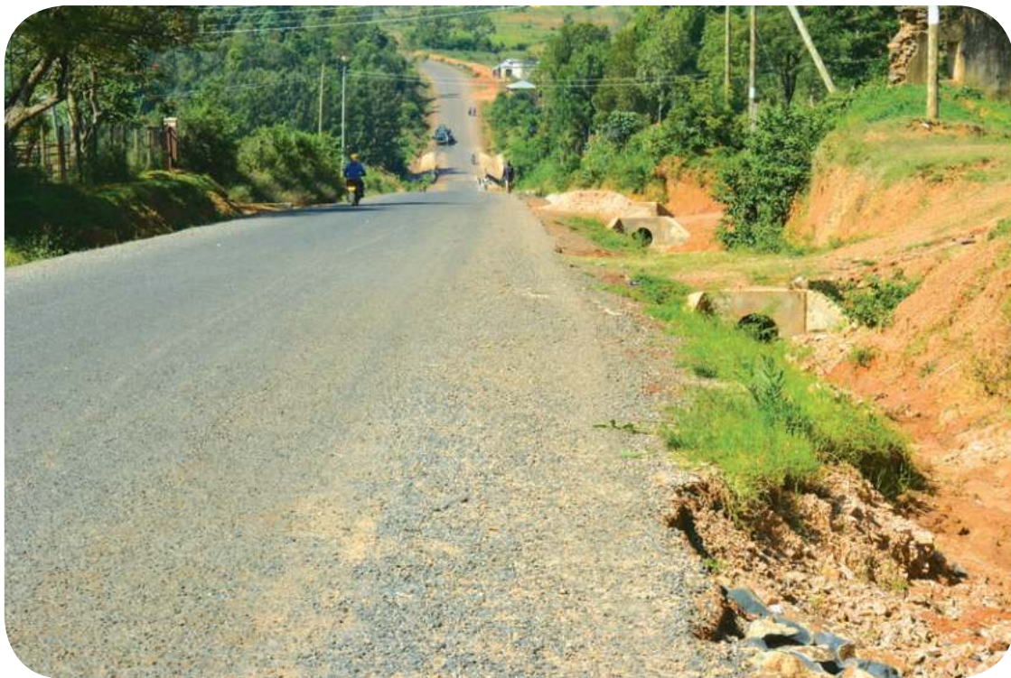
Luanda-Ekwanda Road upgraded to low volume seal Standard
