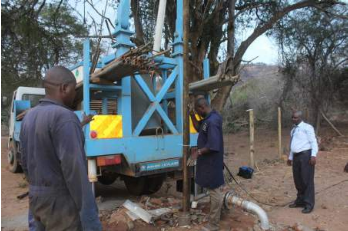
Drilling of Boreholes
